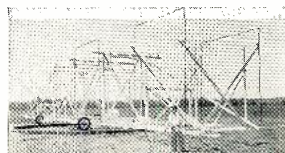
Directional antenna used by Karl G. Jansky in discovery of stellar radio signals at Bell Telephone Laboratories in 1932.
